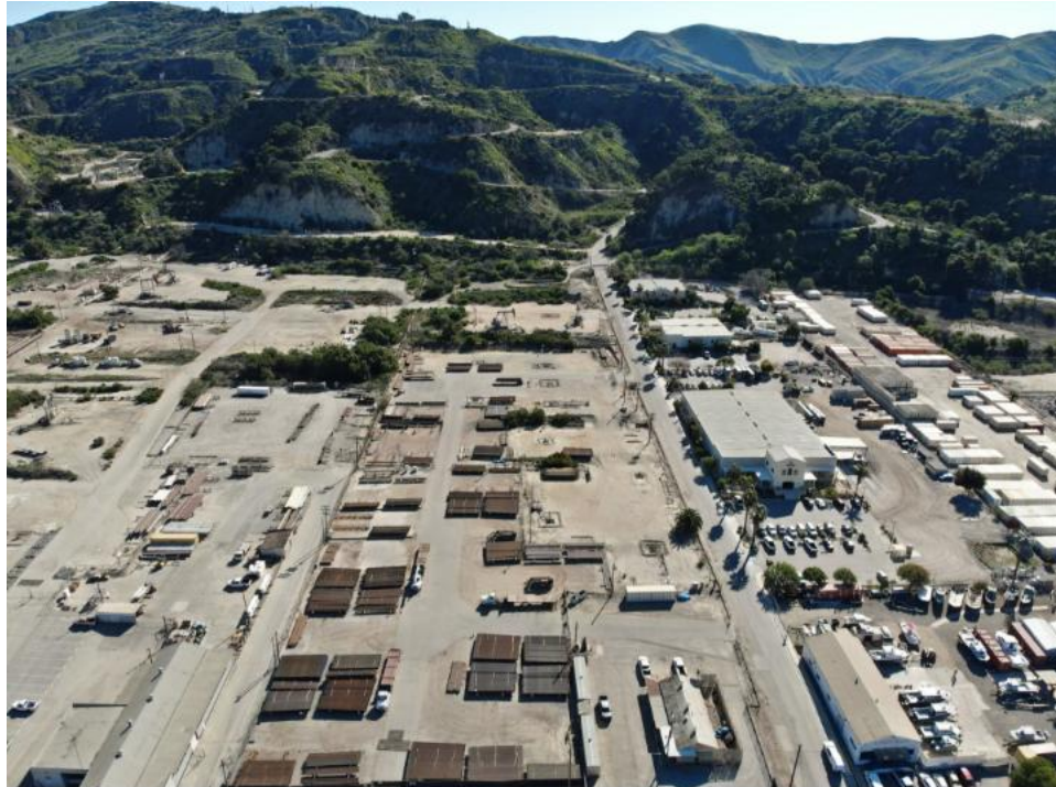
Exhibit 3-26: East-facing view of the Ventura Steel Site
