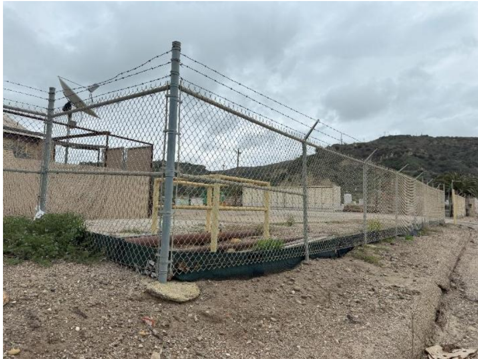
Exhibit 3-16: Existing conditions at the southwest corner of the Ventura Steel Site
