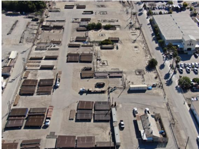
Exhibit 3-30: East-facing view of the Ventura Steel Site
