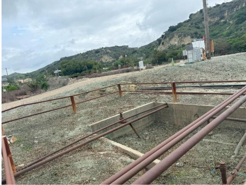
Exhibit 3-13: Existing valve vault on the Ventura Steel Site
