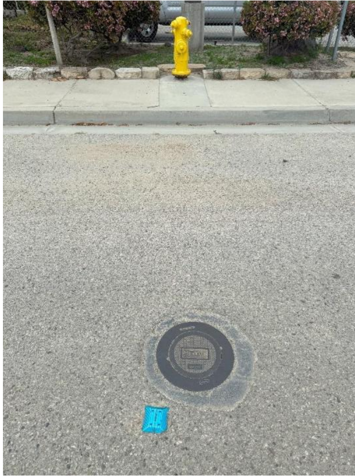
Exhibit 3-11: Fire hydrant on the south side of East Shell Road
