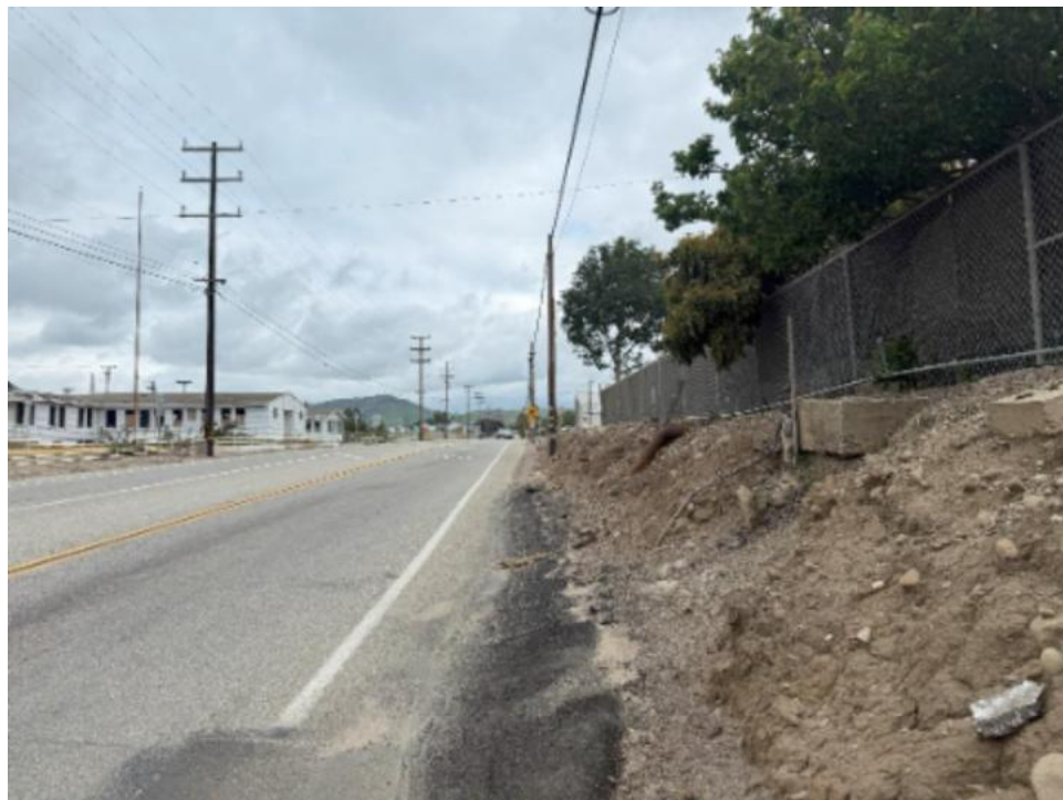
Exhibit 3-34: North-facing view of Ventura Steel Road and connection point for site electrical
