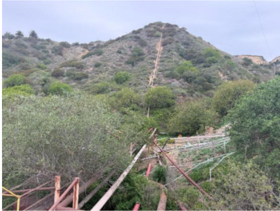
Exhibit 3-33: North-facing view of the Ventura Steel Pipeline Alignment from School Canyon Road
