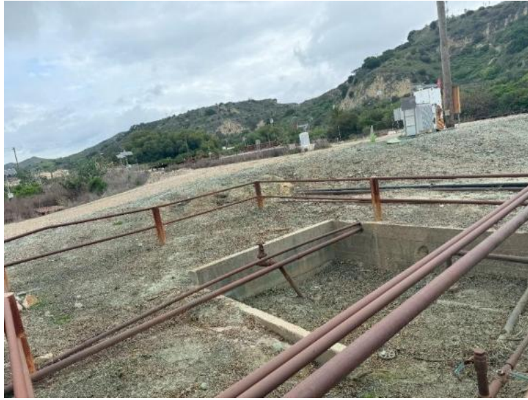
Exhibit 3-29: Existing valve pit at the Ventura Steel Site
