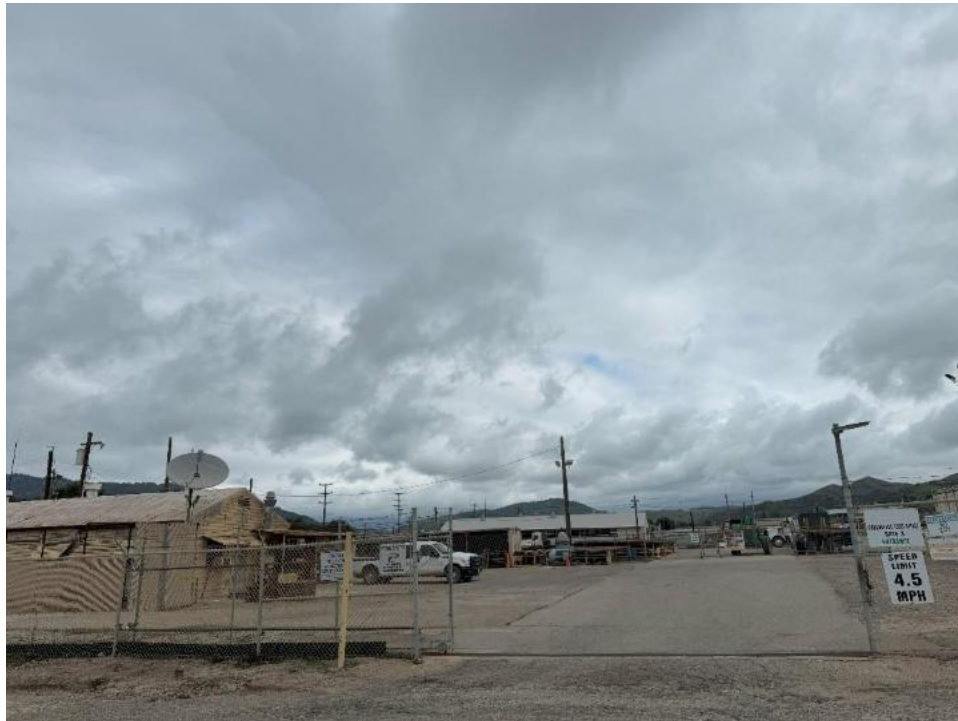
Exhibit 3-19: Existing gate/entryway into the Aera facility at the Ventura Steel Site
