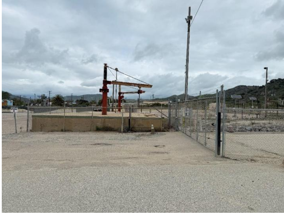
Exhibit 3-22: Existing conditions at the Ventura Steel Site's temporary staging area
