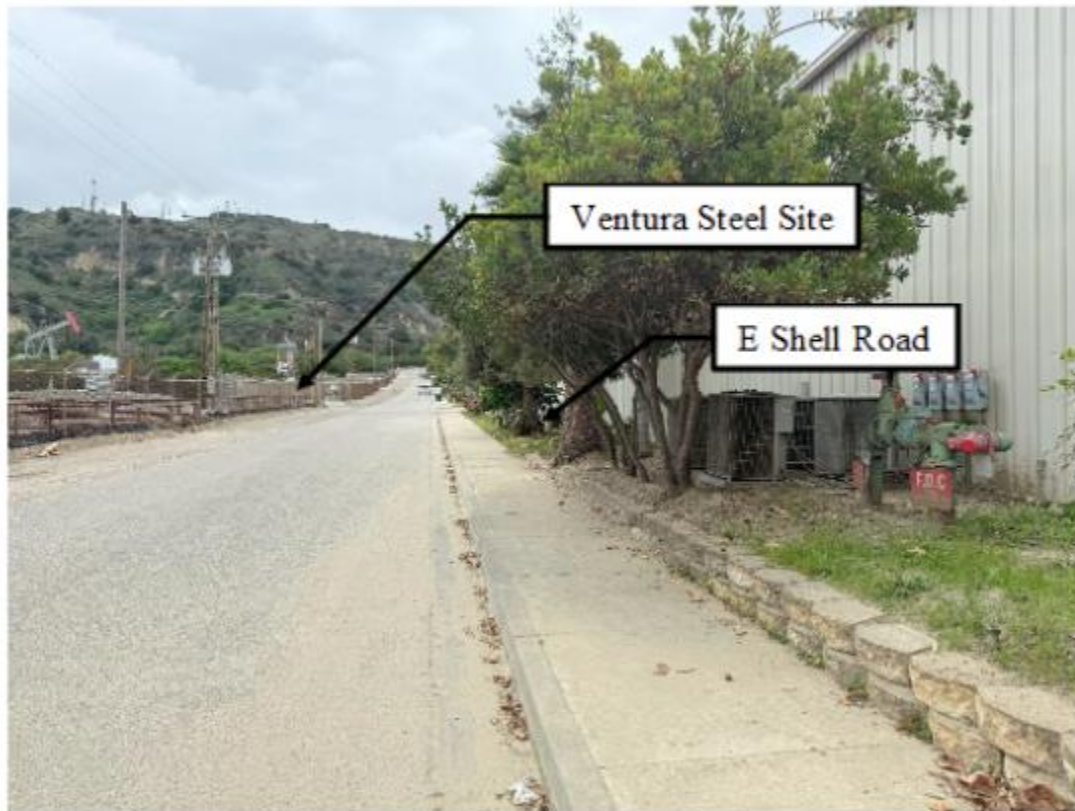
Exhibit 3-12: Fire department connection on the south side of East Shell Road, showing potential fire water main connection
