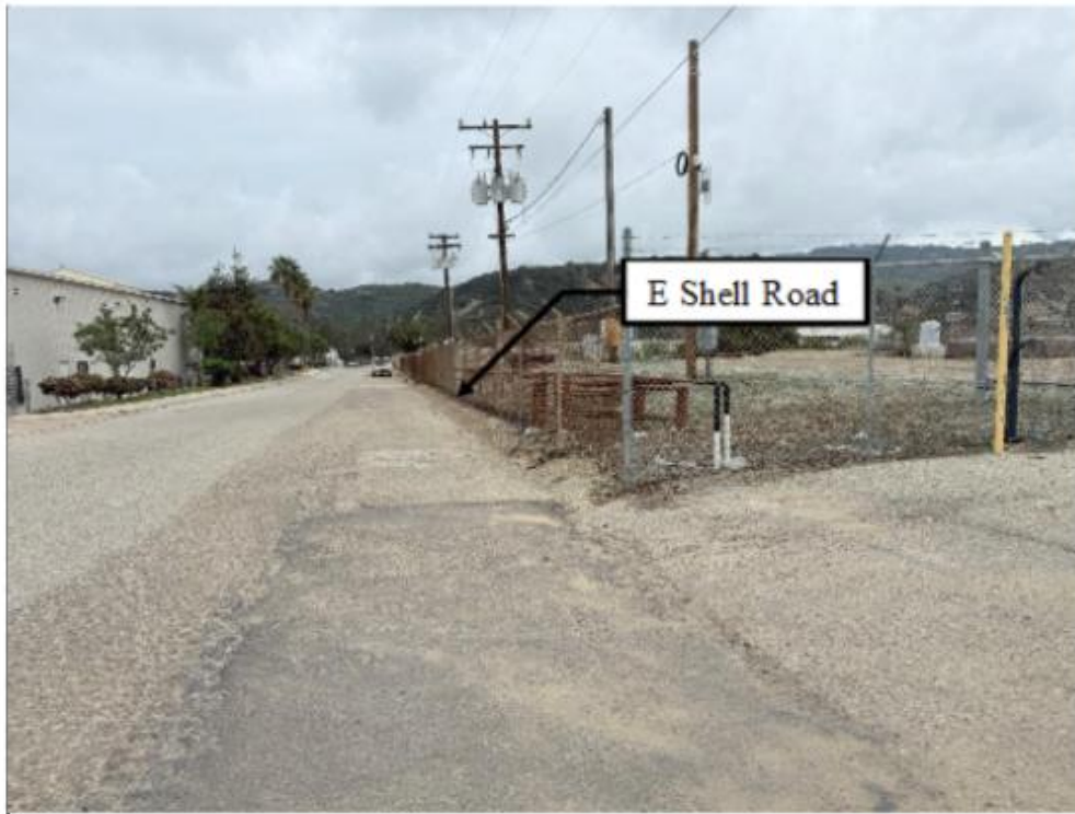
Exhibit 3-5: West-facing view of the existing Ventura Steel Site and East Shell Road
