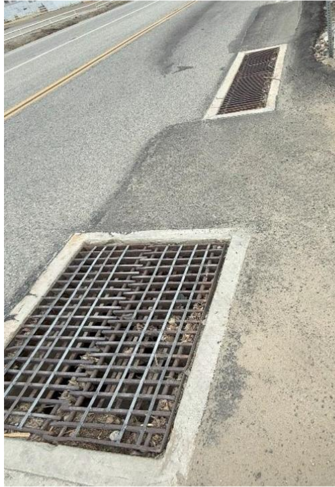
Exhibit 3-17: Storm drain inlets at the intersection of Ventura Steel Road and East Shell Road
