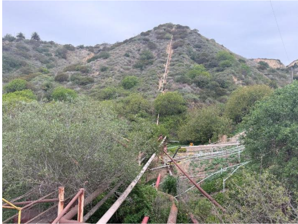
Exhibit 3-2: North-facing view of Ventura Steel Pipeline Alignment from School Canyon Road
