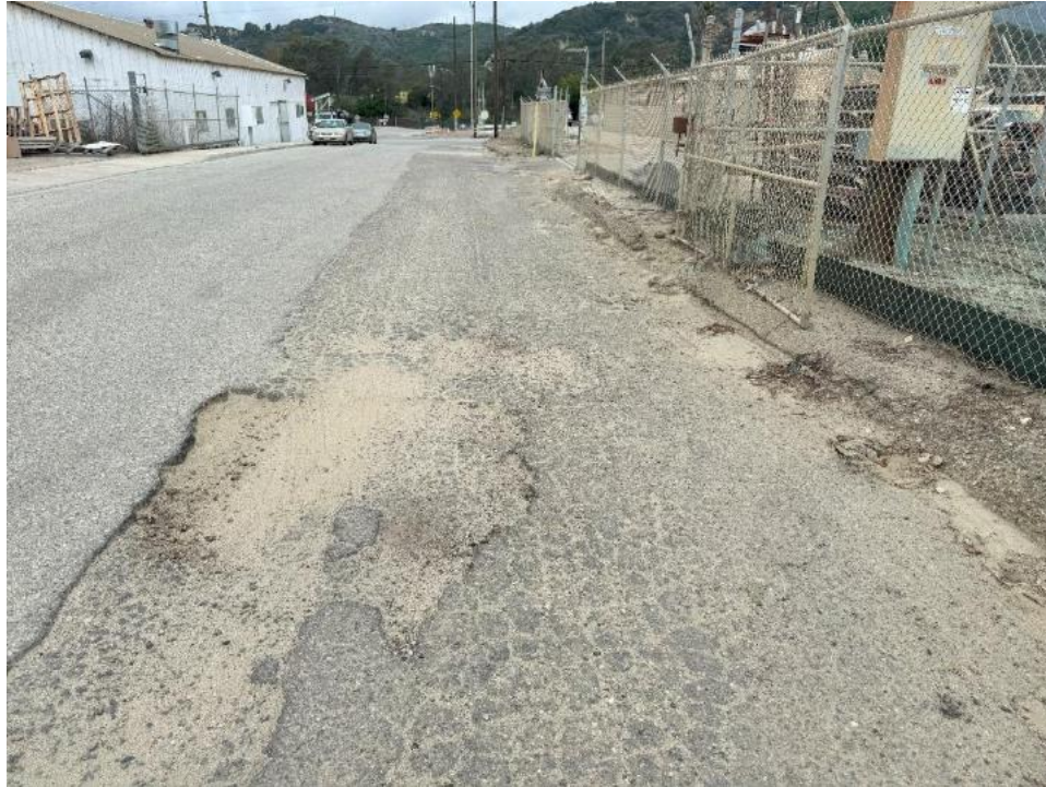
Exhibit 3-10: West-facing view of existing conditions on East Shell Road at the Ventura Steel Site
