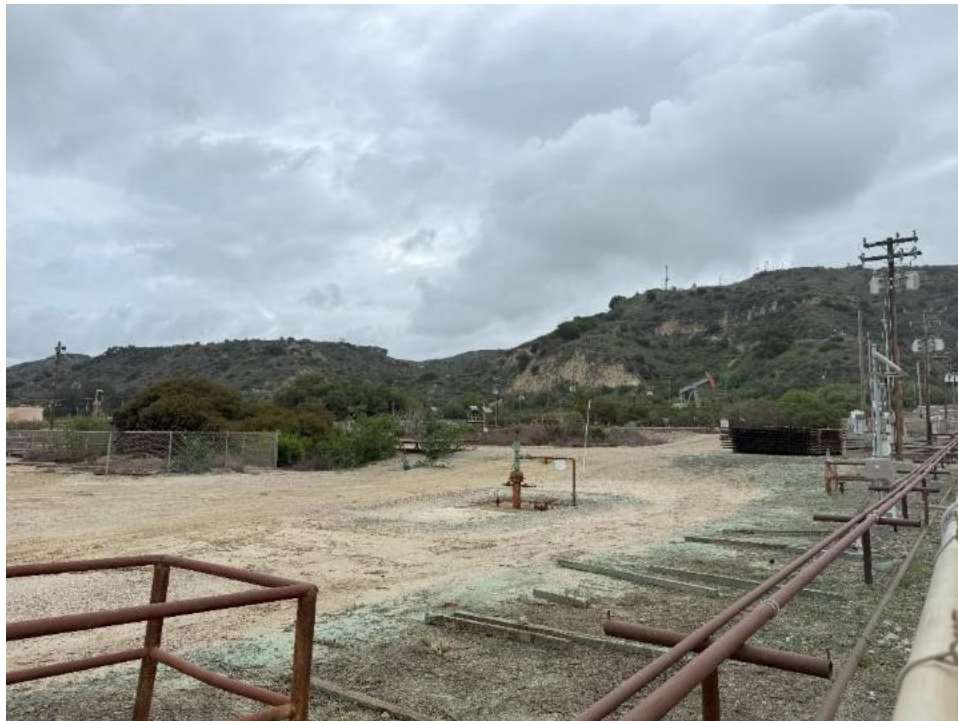
Exhibit 3-7: Northeast-facing view of existing oil wells and associated piping at the Ventura Steel Site
