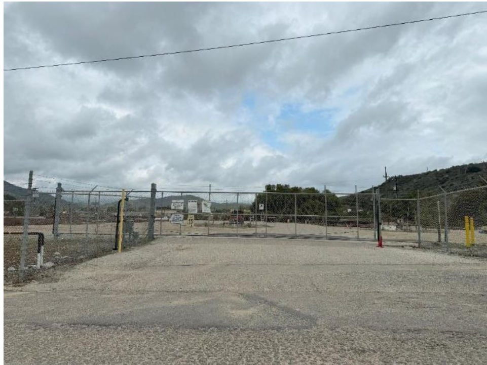
Exhibit 3-3: North-facing view of the gate/entrance to the existing Aera facility at the Ventura Steel Site from East Shell Road
